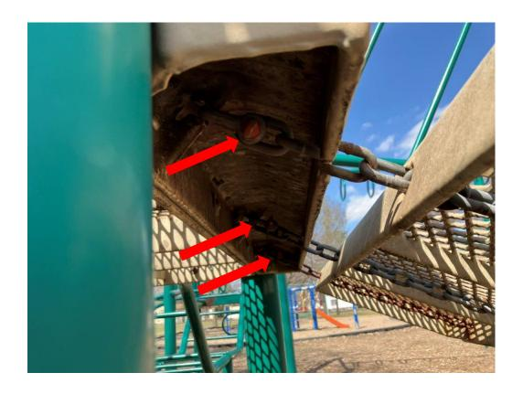
22. The clevises and anchor points for the hanging walkway should be replaced as they are nearly worn through.
