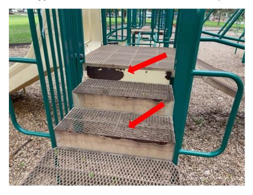
22. The metal of the standing platforms are aging and rusting. Structural integrity of the metal is weakening and is becoming a safety concern.
