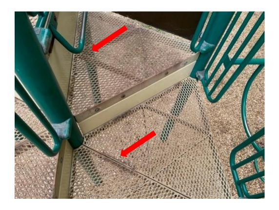
22. The metal of the standing platforms are aging and rusting. Structural integrity of the metal is weakening and is becoming a safety concern.
